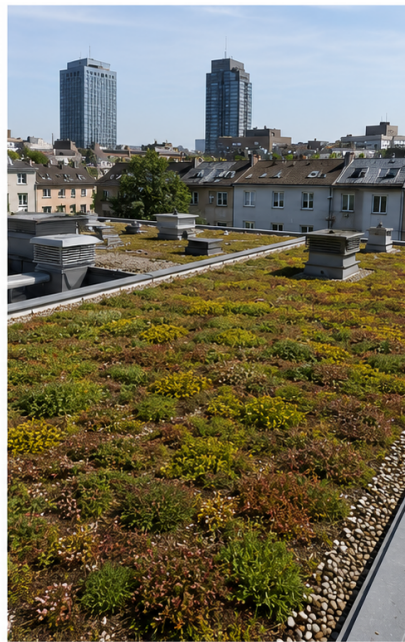
146 roof and facade greening on buildings
