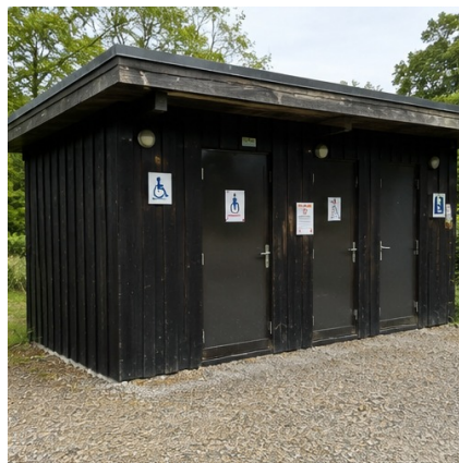
(b) Toilet access
